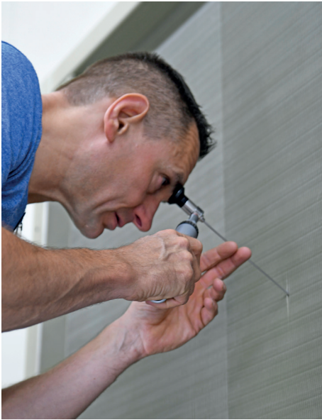
Endoscope inspection between heat exchanger fins
