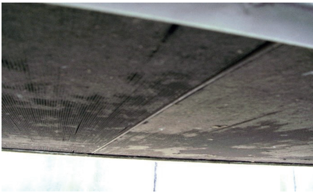
Visible fouling in heat exchanger
